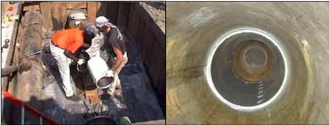
Graph 4.2: Sleeve inserting / Sleeve installed [12]
