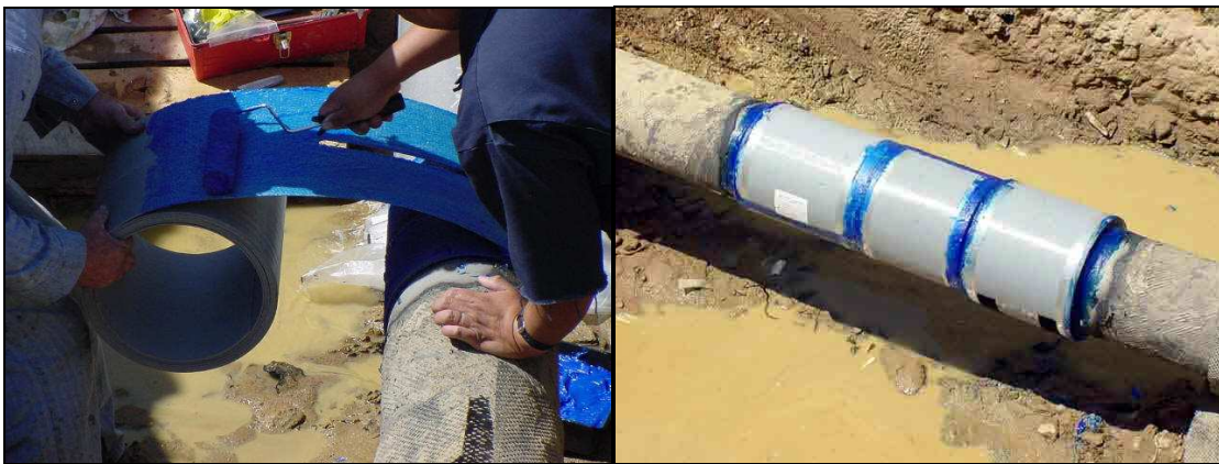
Graph 4.4: Installation of WeldWrap [14]
